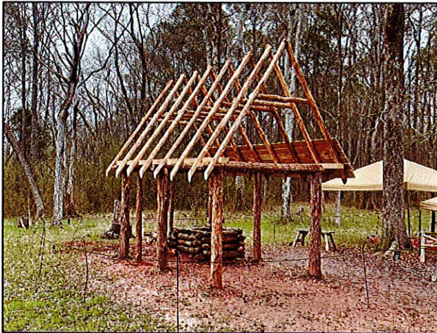
Frame of Blacksmith Shed complete, March 8, 2024
